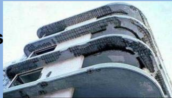
Large spall area on all balconies of building [Photo Credit: Robert Pirro]
