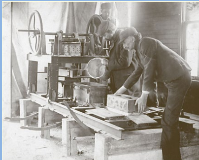
Making Concrete Blocks 1904
