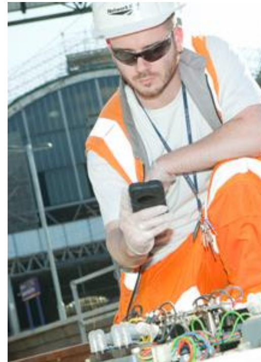
Picture courtesy Network Rail
