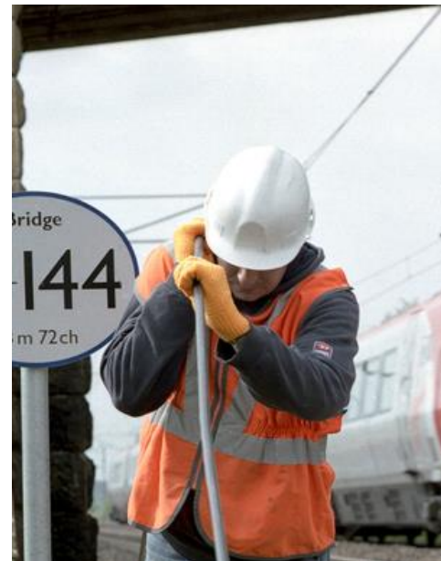
Picture courtesy Network Rail
