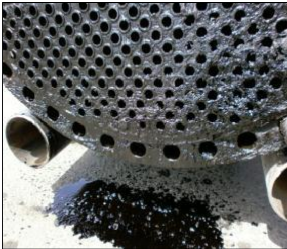
Sludge from Heat Exchanger
